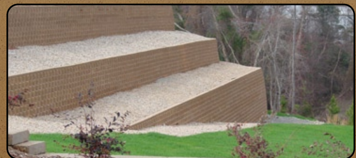
CONCRETE RETAINING WALLS
